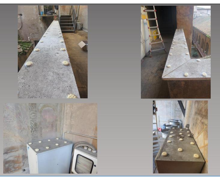
The ledges and air conditioning equipment inside the inner courtyard were treated with dishes of 小島 *Bird Free* as shown above.
