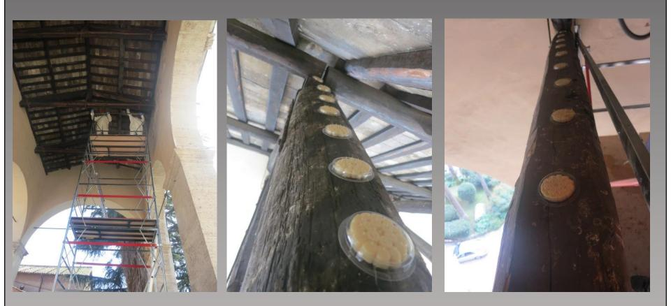
The seven delta-shaped rafters in the south section of the loggia were first cleaned. Dishes of 小島 *Bird Free* were then fitted to the upper parts of the rafters at 20cm centres (above middle), and to the lower part of the rafters at 25cm centres (above right). The dishes are invisible from below.
