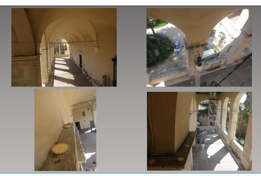
Dishes of 小島 Bird Free were fitted at 25cm centres to all small ledges on both sides of the L-shaped loggia to prevent displacement.
